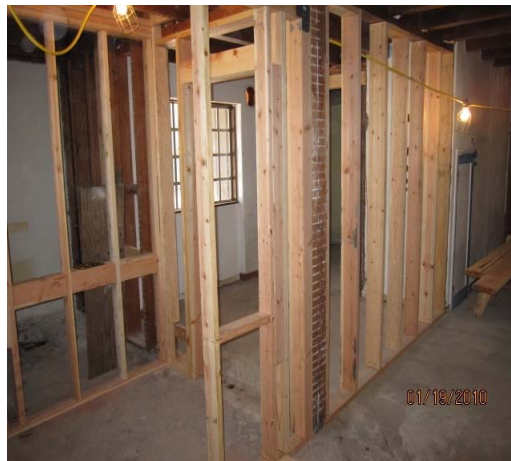
Interior Wall Framing
